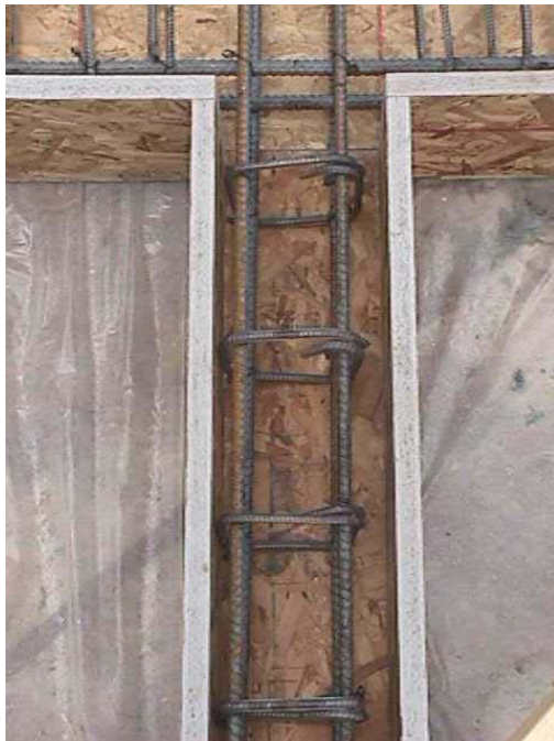
Figure A. 4 Typical stirrup spacing of the column
