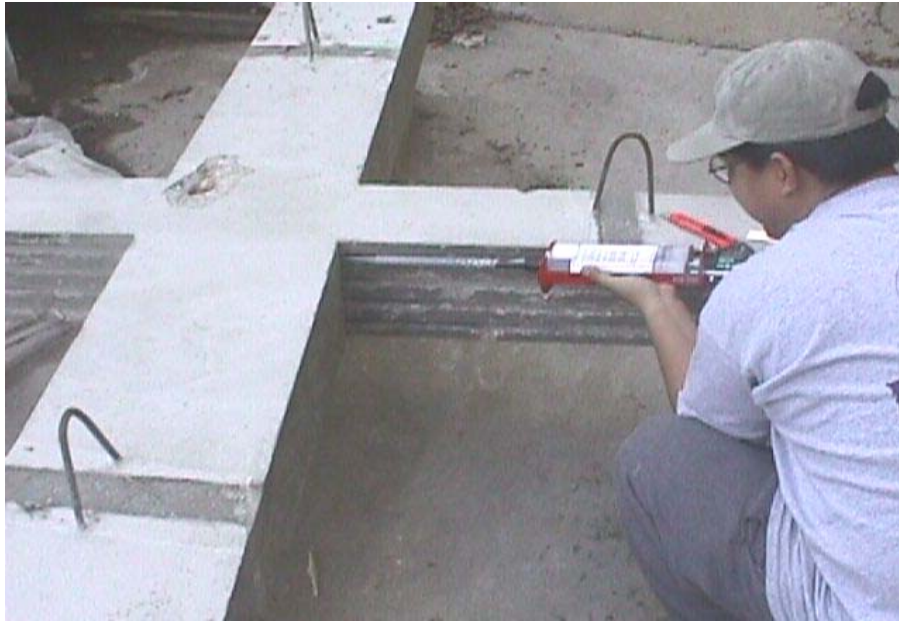
Figure A. 19 Pouring of the first layer of concrete paste into the grooves
