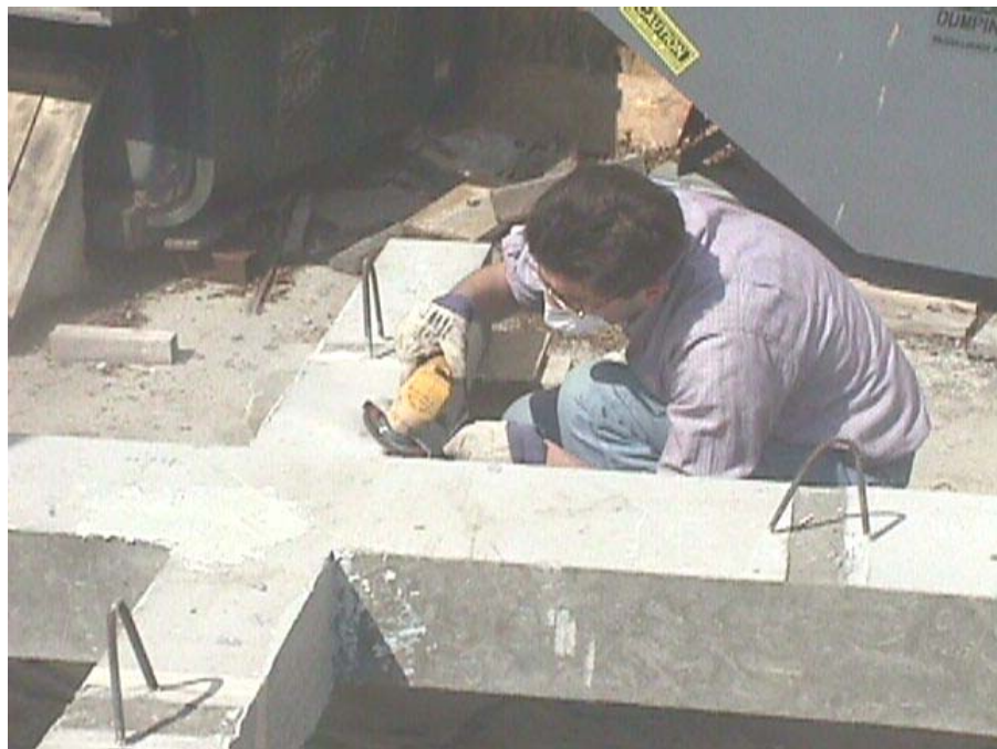
Figure A. 10 Rounding of the corners prior to laminates application
