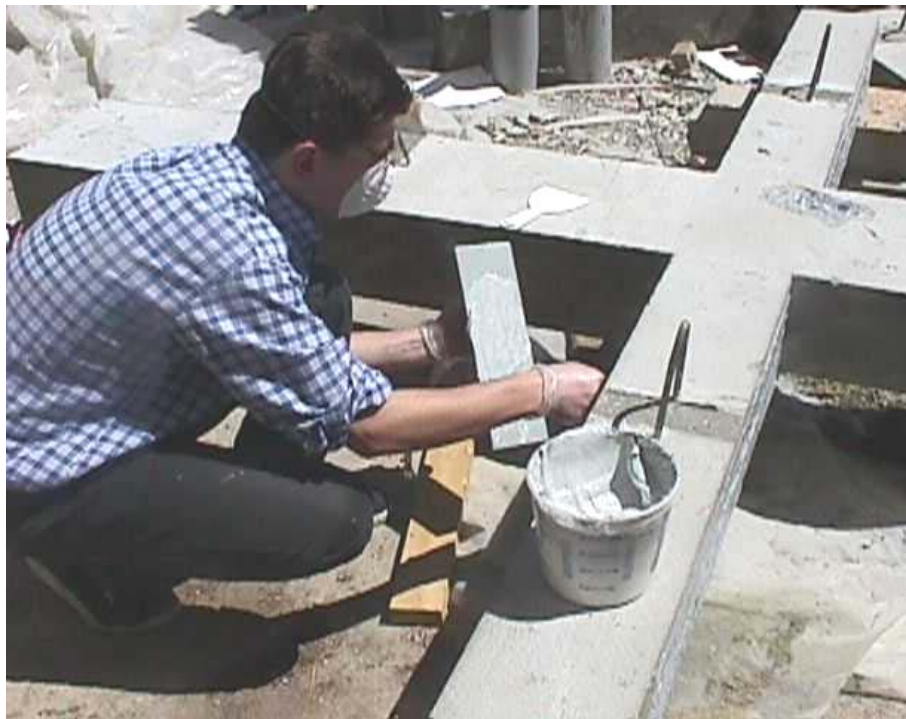
Figure A. 22 Finishing of the surface after installation of NSM rods
