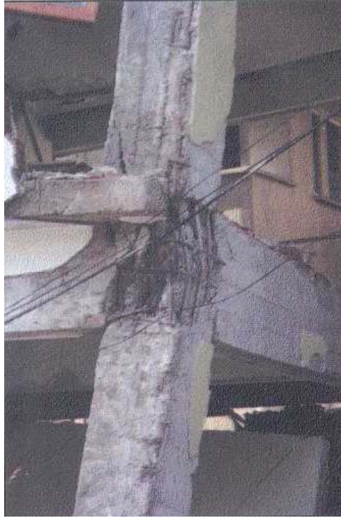
Figure 1. 2 Failure of an exterior joint
