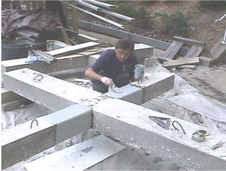
Figure A. 13 Filling of holes and imperfections by putty
