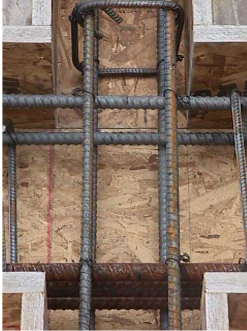
Figure A. 3 Typical metallic reinforcement of the nodal zone
