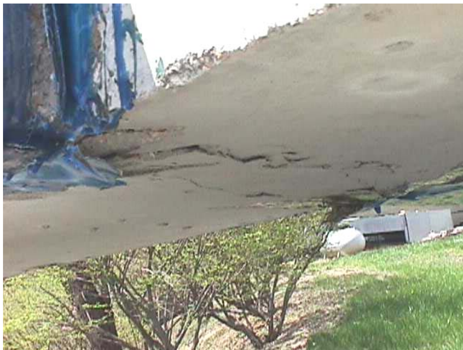
Figure B. 32 View from the bottom of panel damage: joint H2
