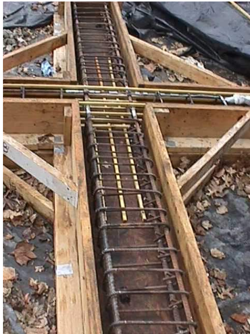
Figure A. 6 View of the beam prior to concrete casting: L4
