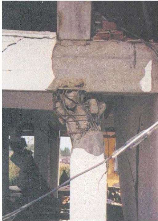
Figure 1. 3 Weak column-strong beam construction
