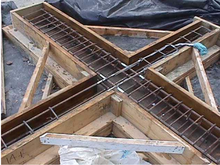
Figure A. 7 Induced confinement defect in the column: H2U
