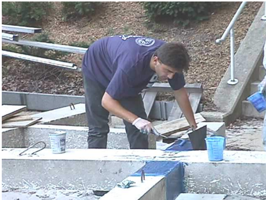
Figure A. 14 Impregnation of fibers by saturant
