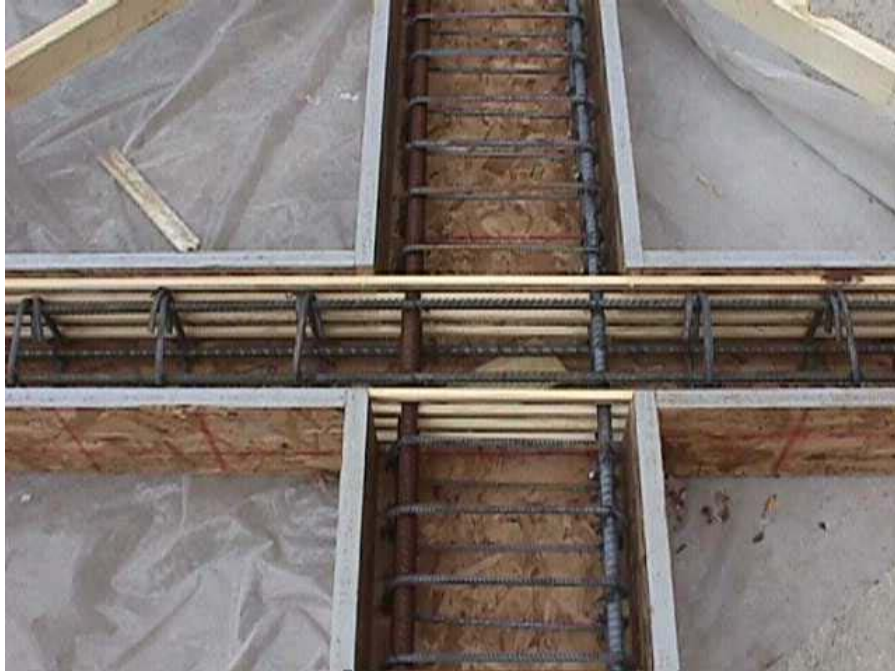
Figure A. 5 Wooden predisposition for NSMR: L3, L4, H3, H4, H5, M3
