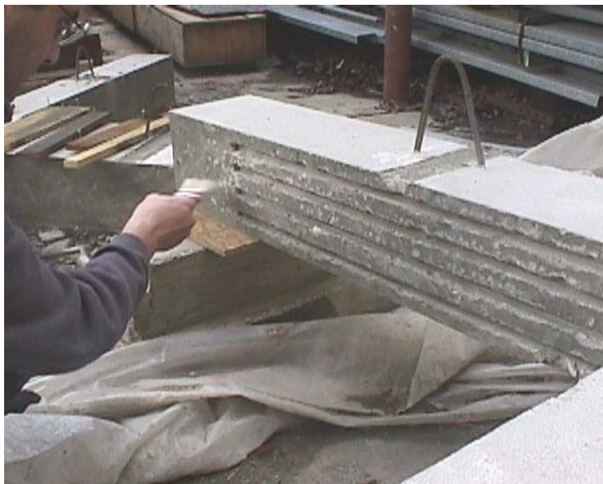
Figure A. 18 Hand cleaning of the grooves
