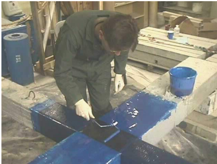
Figure A. 26 Application of carbon laminate as vertical reinforcement of the panel
