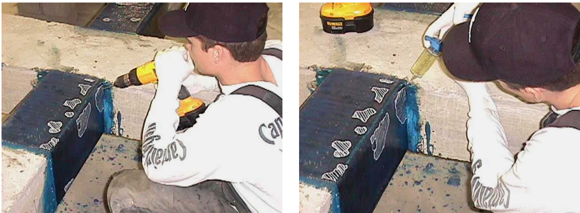
Figure 3. 10 Primer injection of bubbles by a syringe
