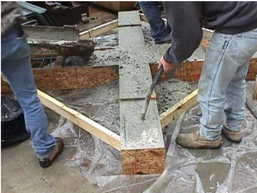
Figure A. 8 Concrete vibration: H1
