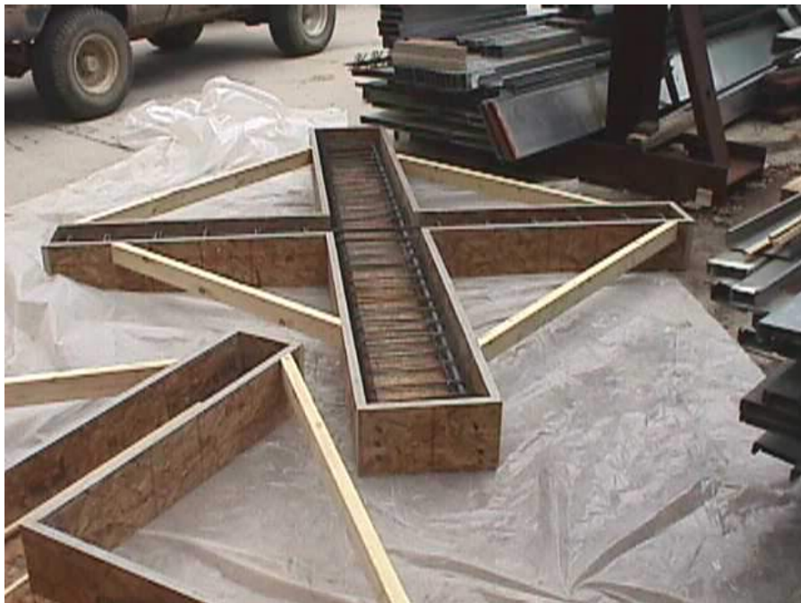
Figure A. 2 Typical beam reinforcement
