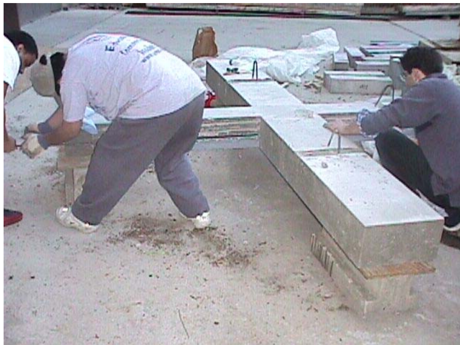
Figure A. 20 Installation of NSM FRP rod
