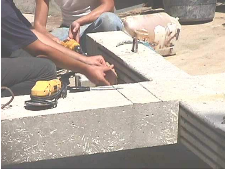
Figure A. 15 Drilling through the panel prior to installation of NSM rods
