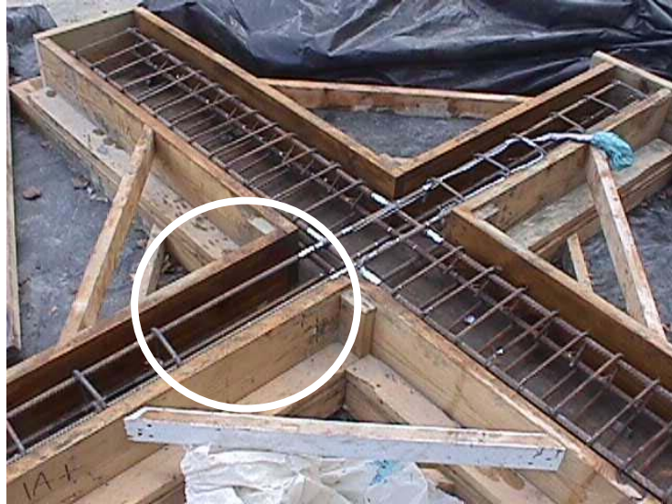
Figure 5. 4 Confinement defect on the superior column of connection H2U
